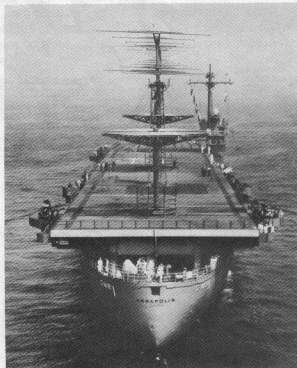
Antennas have replaced a once vital and busy World War II flight deck.
