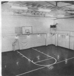
The VLF transmitter room awaits equipment. Until gear arrives, it makes a fine basketball court.
