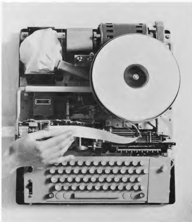
Note the compactness of the keyboard-punch with the lid off, and how easy it is to replace the tape. You merely slip it into the tape holder and thread it through the punch.
