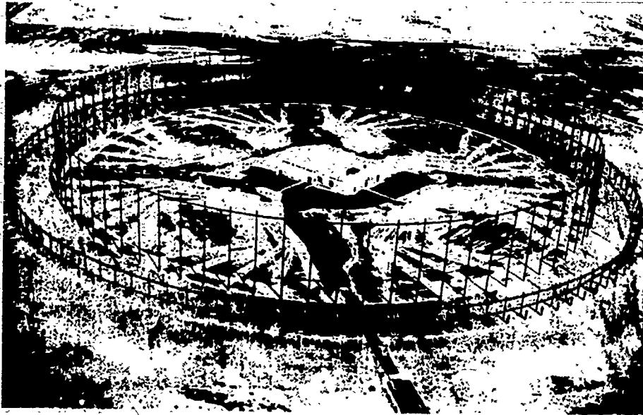
Figure 7-34.—Circularly disposed antenna array (CDA).
