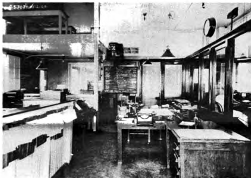
CONTROL DESK AT NBA, BALBOA IN MAY 1929. FOR A TIME I RELIEVED HAROLD CRAIG (SOWP 308-SGP) AS CONTROL OPERATOR. TWO TELETYPE ARE IN THE SETBACK OF THE WALL COUNTER - ONE TO PORT CAPTAIN AND ONE TO PANAMA TELEGRAPH OFFICE. ON THE MEZZANINE WE HAD SPACE FOR SHORT WAVE SPECIAL OPERATIONS WHEN FLEETS WERE IN THE VICINITY ON MANEUVERS OR WHEN THE ARMY HAD A HOT-SHOT DRILL BEHIND THE GLASS PANELS TO THE RIGHT WERE THE SHIP OPERATORS (COMM'L AND NAVY CIRCUITS) THE LONG WAVE RECEIVERS FOR THE FLEET BROADCASTS, THE NSS CIRCUIT AND THE NAZ CIRCUIT TO MANAGUA WITH THE MARINE CORPS SANDINO HUNTERS. THE TELEGRAPH CIRCUITS, 5 OR 6 OF THEM, CAME TO THE CONTROL DESK TO THE SWING-ARM SOUNDERS.
