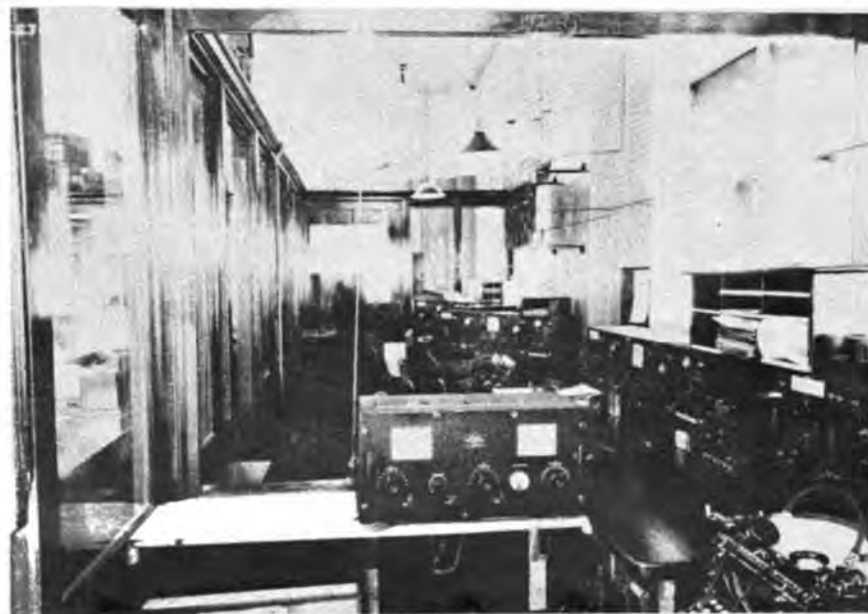
NBA, BALBOA, OPERATING POSITIONS LOOKING NORTH IN THE GLASS ROOM. FACING RECEIVER WAS THE MODEL RW, FINAL VERSION OF THE XW DEVELOPED BY COMMANDER WILLIAMS... IT WAS USED ON NSS AND THE SE143 VERY LOW FREQUENCY RECEIVER, NOT VIIBLE, WAS FOR THE NAS' ARCS.
