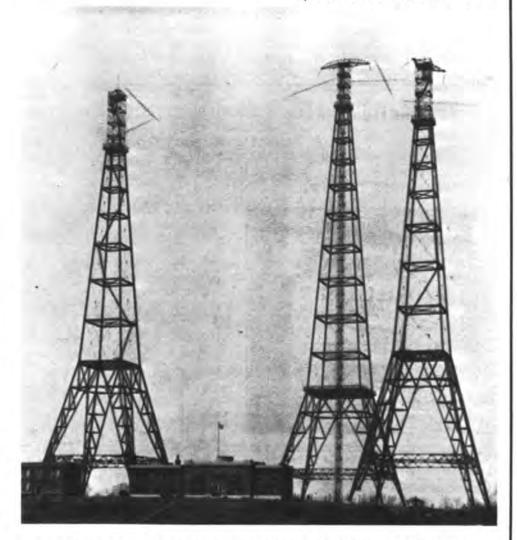
UNITED STATES WIRELESS STATION AT RADIO, VIRGINIA, HAVING DIRECT COMMUNICATION WITHIN RADIUS OF OVER 3000 MILES -- TALLEST TOWER IS 600 FEET HIGH AND THE OTHER TWO, 450 FEET EACH. Photo - U.S. Naval Photographic Center
