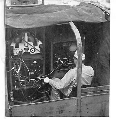
The 1B mounted in a USMC 6x6 truck, showing position of operator and equipment.
