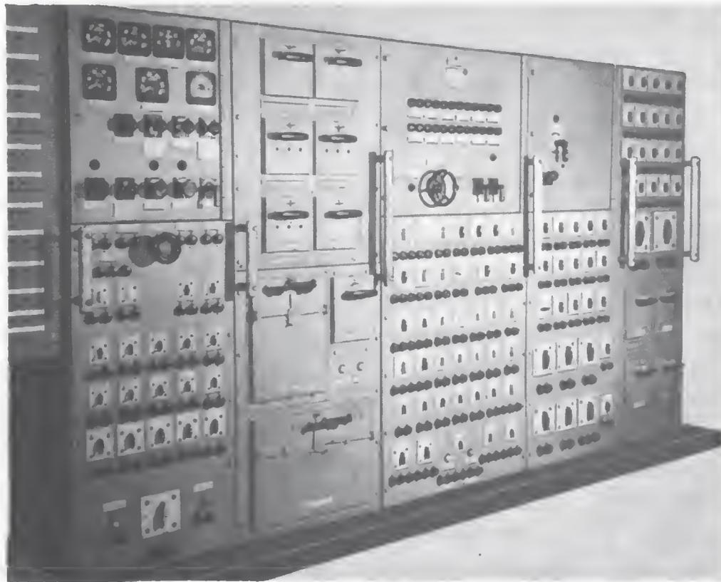
Figure 2-2.—Dead-front I. C. switchboard.
